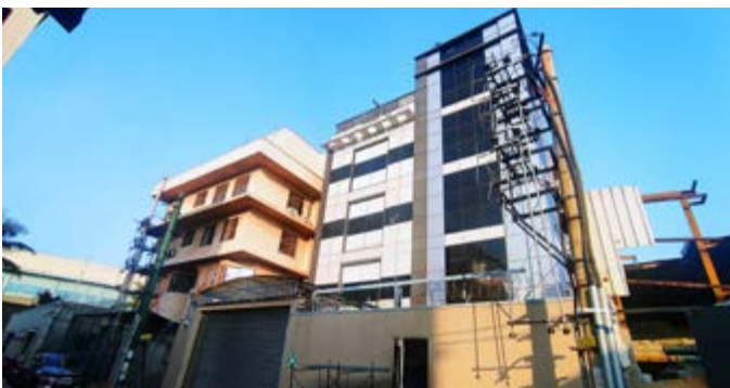
State-of-the-art RFID unit in Bengaluru that houses our R&D center
